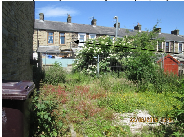
Rear elevations of houses on Gordon Street
